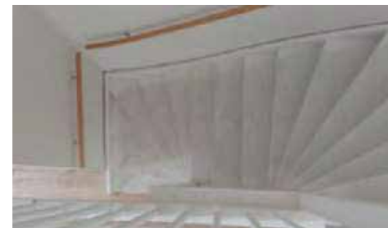
Trap In grondverf.
